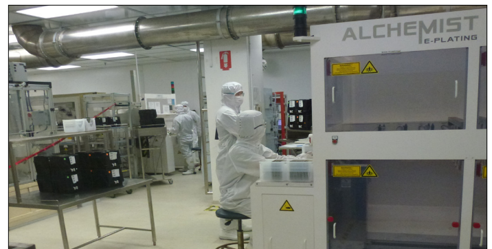
HP's Printhead Electroplating Facility
